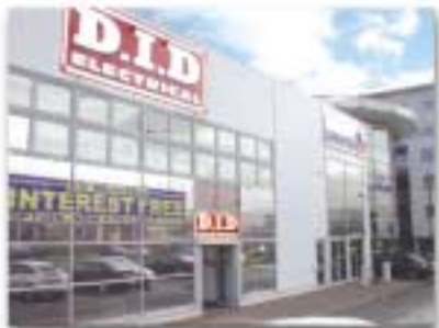
DID Electrical, Belgard Road
